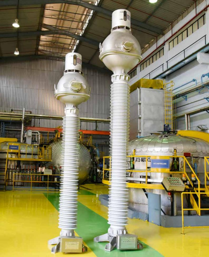
245kV and 420kV 50 / 63 kA 3000A Current Transformers with Polymeric Insulators Developed by CG at its Manufacturing Facility in Nashik
