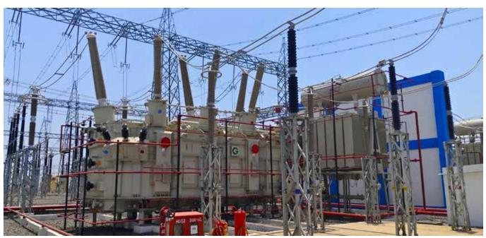
500MVA 400kV 3-Ph ICT Supplied by CG for Agar Malwa Substation Project
