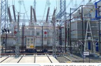
500MVA 400kV 3-Ph ICT Supplied by CG for Karur Substation Project
