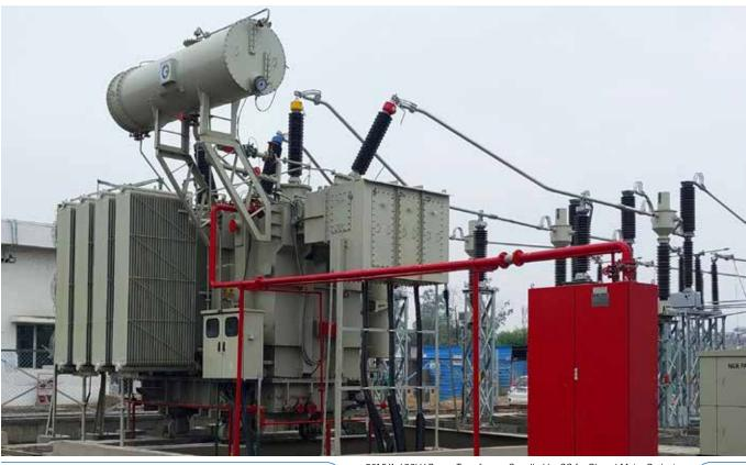
50MVA 132kV Power Transformer Supplied by CG for Bhopal Metro Project
