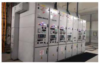
33kV GIS Supplied by CG for Underground Substation, UPMRCL, Agra Metro Project
